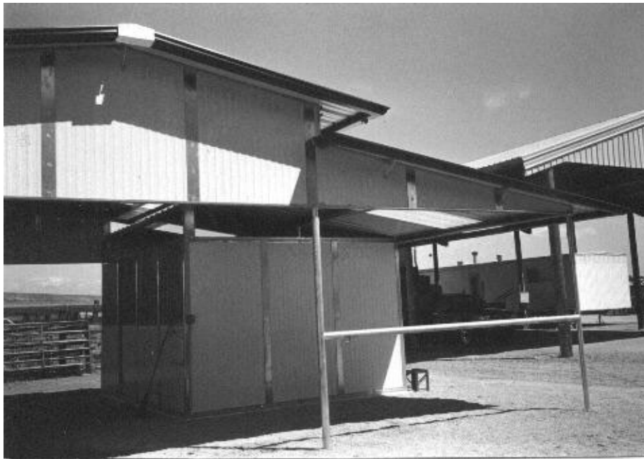
GABLE ROOF—RAISED BREEZEWAY WITH ROOF EXTENSION
