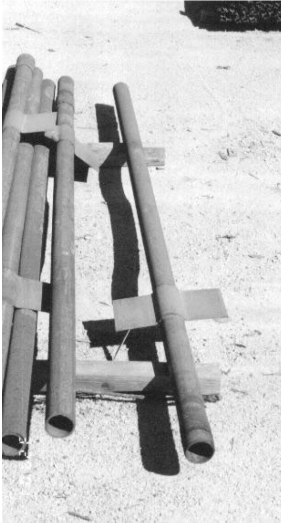
Steel end post with spade
