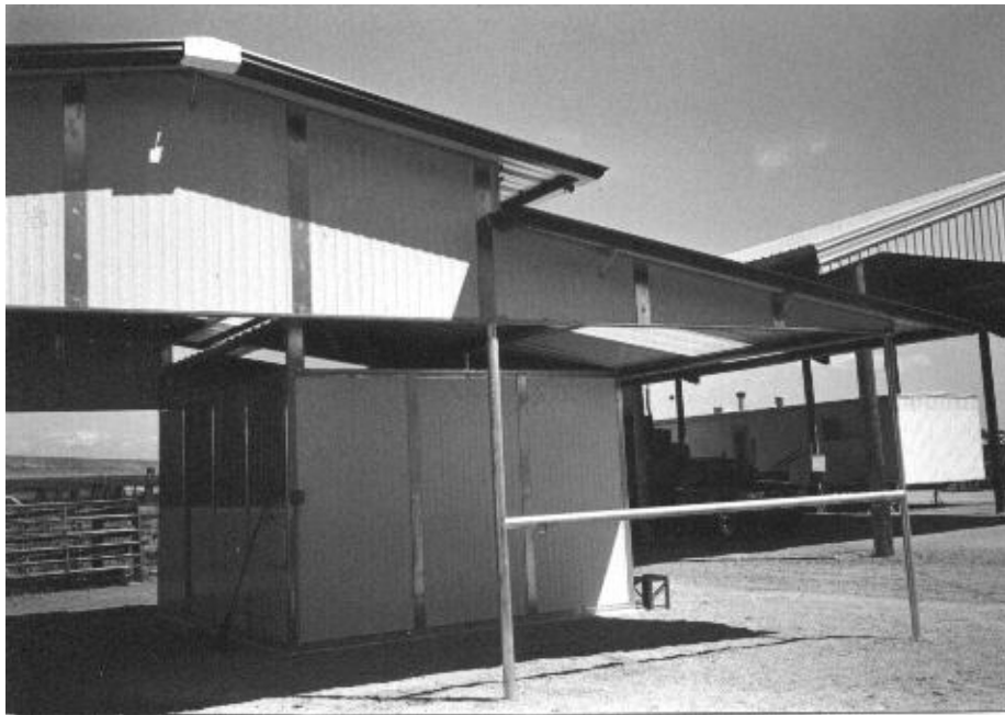
GABLE ROOF—RAISED BREEZEWAY WITH ROOF EXTENSION
