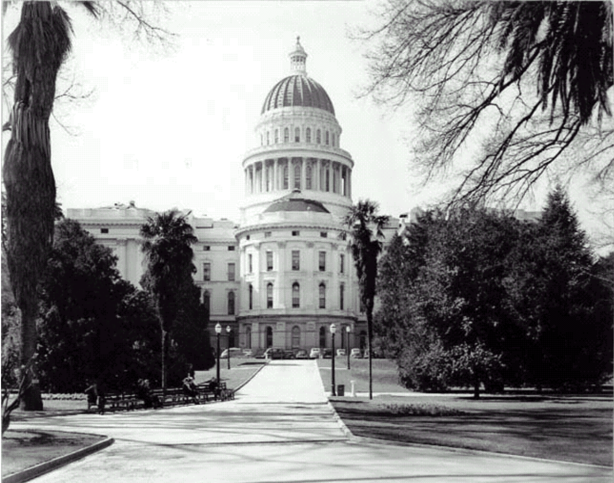
State Capitol Building (from the East) c.1945 Photo courtesy of California State Archives
